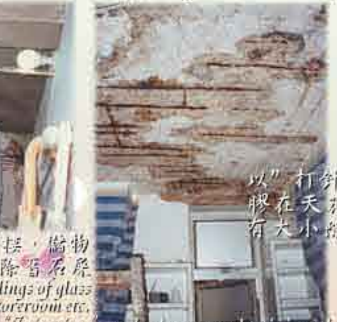
以"打針"形式注入 Tacss 020-NG 防水膠在天花牆隙內自動起泡膨脹充塞所有大小縫隙，達致防漏及防水效果。 "Injection" method was used to inject the Tacss 020-NG waterproof glue. It will automatically be bubbled and enlarged to block all the large and small gaps so as to enable the leakage prevention and waterproof effect.
