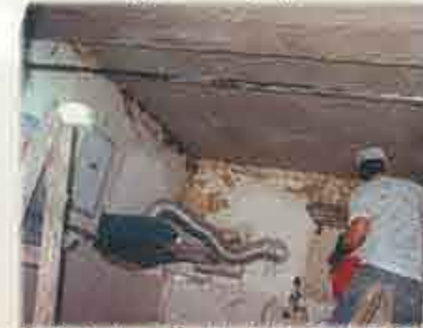
玻璃隔房、動物沖涼室及寫字樓、儲物室等屋內各處天花頂全部去除舊石膠 Remove the old concrete layer at the ceilings of glass cat room, animal bathroom, office and storeroom etc.
